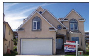
115 Signature Terrace S.W.
