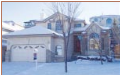
123 Patterson Drive, SW $439,900 DRAMATIC 2 STOREY, QUIET STREET
