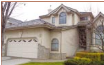
123 Patterson Drive, SW $439,900 DRAMATIC 2 STOREY, QUIET STREET
