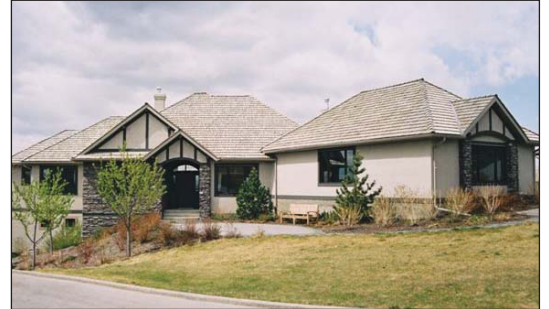
29 Slopes Road S.W.
