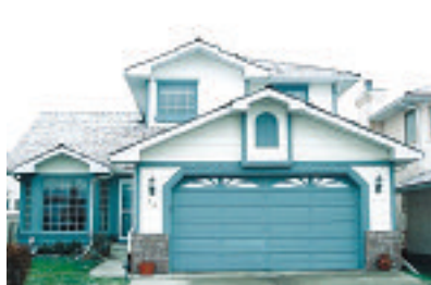
56 Douglas Woods Grove, SE
