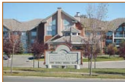
Richmond Hill, $498,000 #324, 6868 Sierra Morena Boulevard, SW
